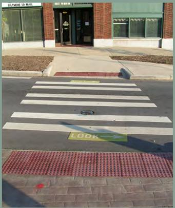
Figure 31—Example of walkway, rumble strips, and return curbing
