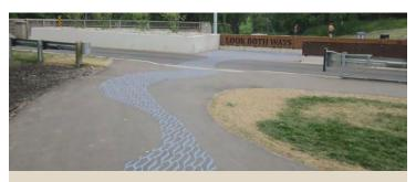
Figure 20—Inlaid Pavement Markings on Pathway & Street, Toronto, ON
