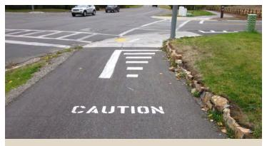
Figure 18—Pathway Approach to Signalized Intersection, Ketchum, ID
