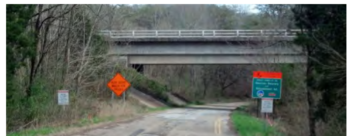
Figure 14—Current Foothills Parkway terminus
